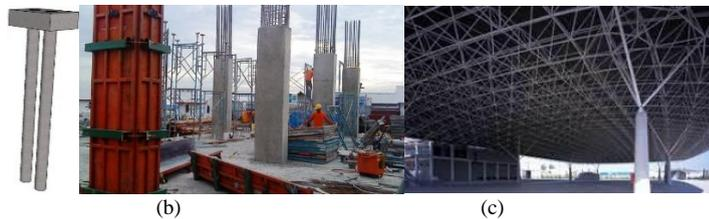
Gambar 11 contoh gambar : (a) Struktur Gambar 1 Pondasi Bore Pile, (b) Beton Bertulang, (c) Rangka *Space Frame*
