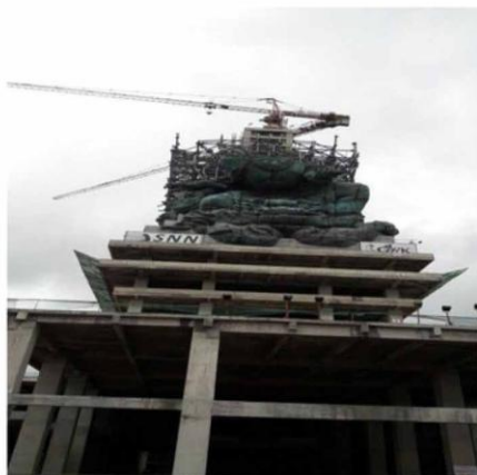
Figure 1 The full statue of Garuda Wisnu Kencana under construction
