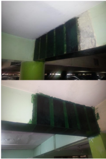
Figure 5. FRP strengthening of beam on first floor.
