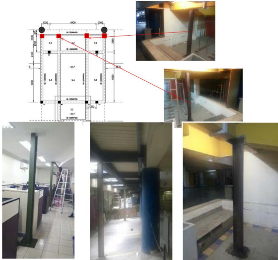
Figure 4. Temporary strengthening of the basement floor
