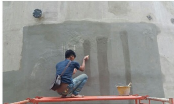
Fig. 8. Waterproof coating on the wall.
