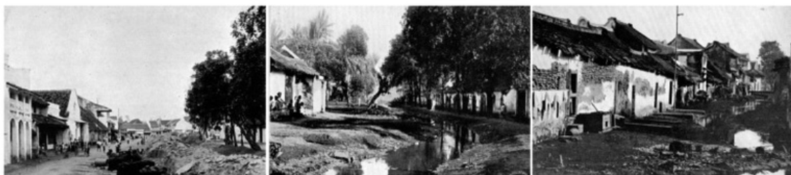
Figure 2: Bacin River before it was turned into Merdeka Street (left & center) and excavation work prior to Merdeka Street (right)
