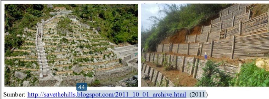
Figure 11. Retaining Wall Illustration to Overcome Landslides
