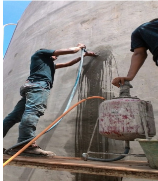
Fig. 7. Leakage injection using cement material with modified polymer.
