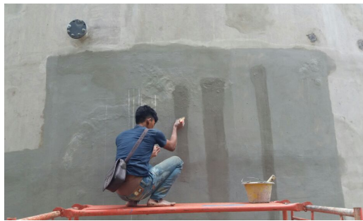
Fig. 8. Waterproof coating on the wall.
