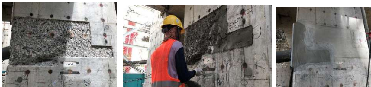
Figure 2. Honeycomb from 10 mm up to 10 mm upto less than 50 mm and concrete cover less than 40 mm
