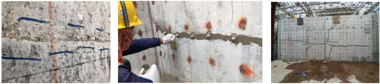
Figure 5. Repair work cold joint and cracks
