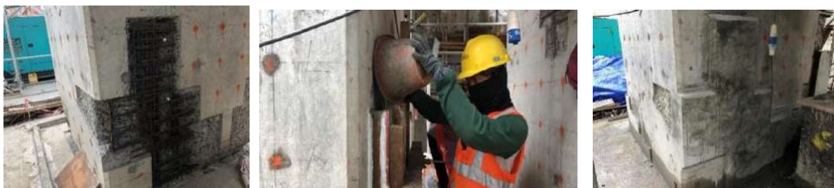
Figure 3. Honeycomb from 50 mm up to 100 mm
