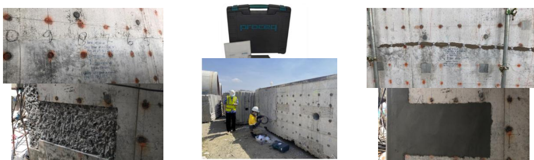
Figure 1. repair work control: before, testing and after work
