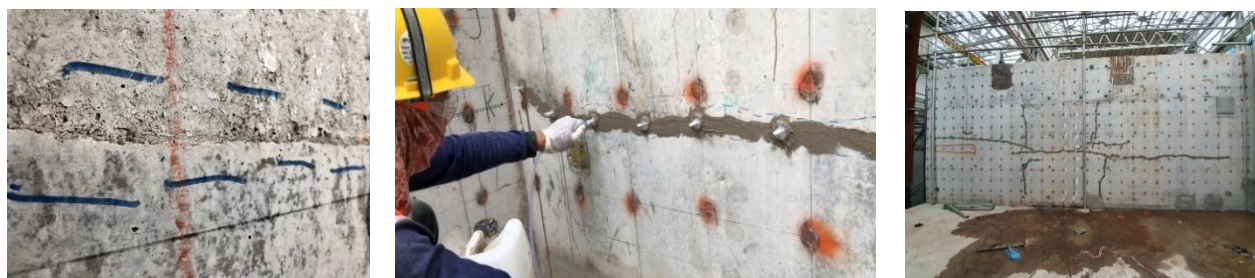
Figure 5. Repair work cold joint and cracks
