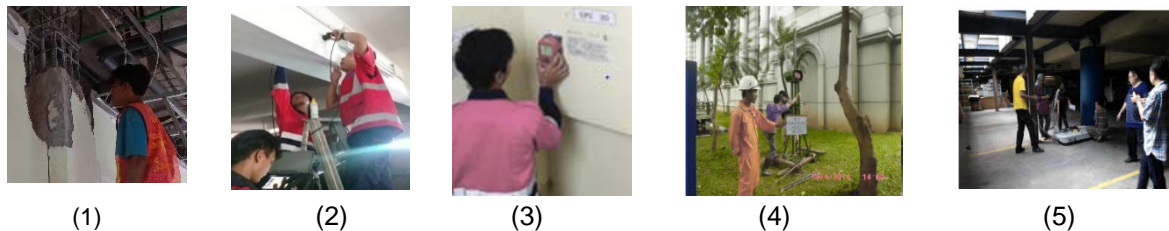
Figure 1. The test is carried out (1) visual observation. (2) UPV. (3) profometer. (4) CPT (5) GPR
