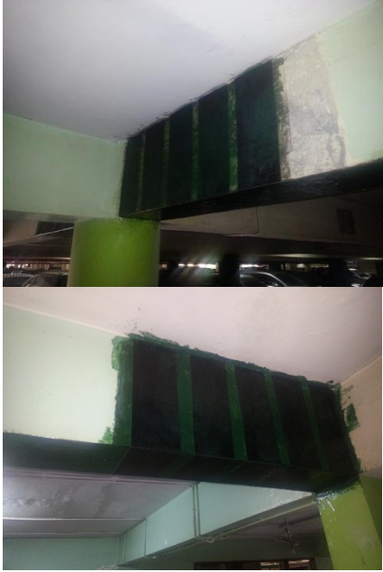
Figure 5. FRP strengthening of beam on first floor.
